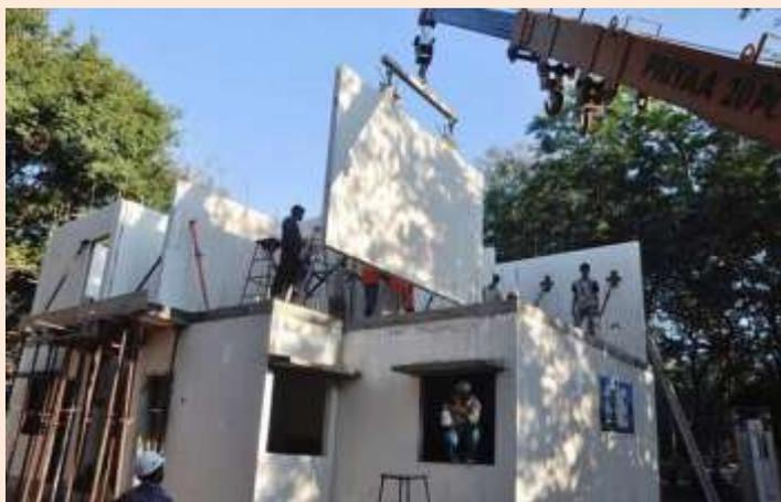
A house being built with Glass Fibre Reinforced Gypsum panels on the IIT, Madras campus, in this file photo.
